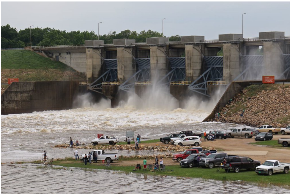
Hugo Dam 2015 Flood
